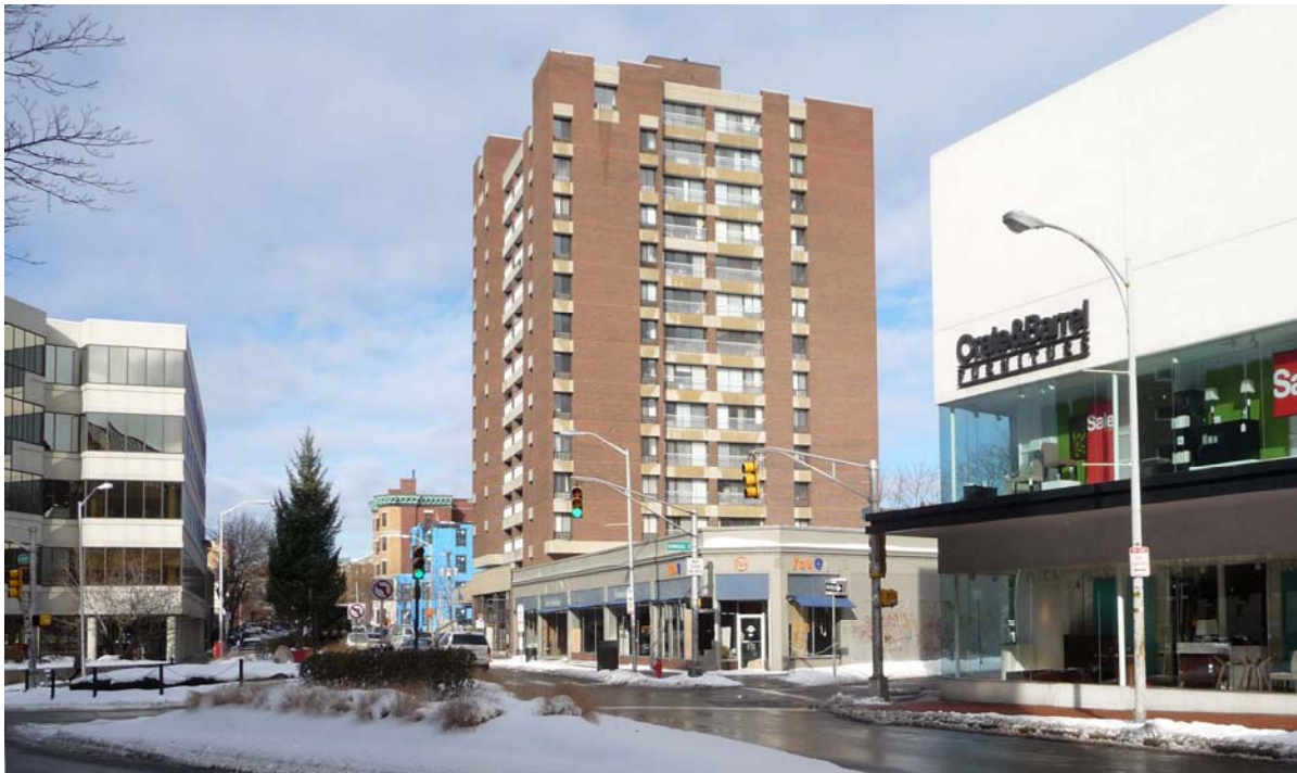
1075 Massachusetts Avenue (center); 1100 Massachusetts Avenue (left); 1105 Massachusetts Avenue (rear); and 1045 Massachusetts Avenue (right). CHC photo, 2010
