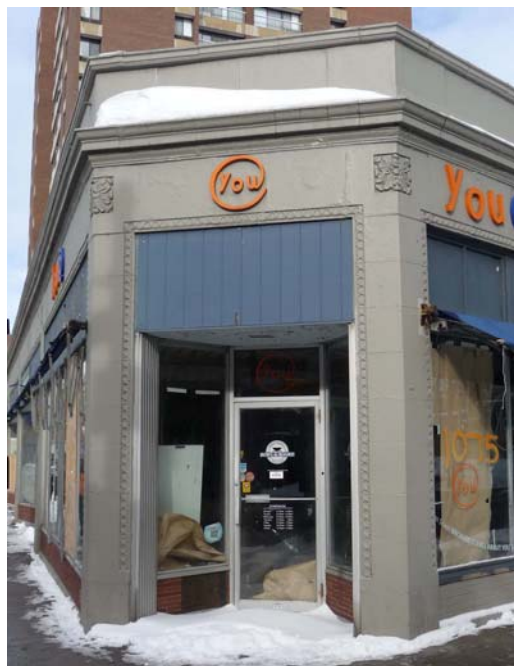
1075 Massachusetts Avenue entrance detail. CHC photo, 2010
