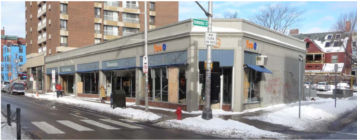
1175 Massachusetts Avenue. CHC photo, 2010.
