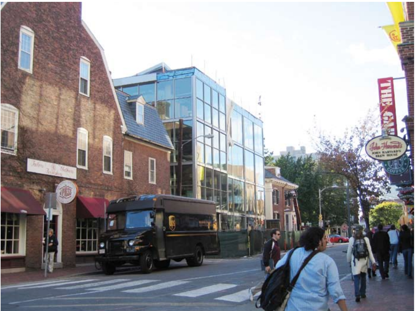
Harvard's 90 Mount Auburn building has a geothermal system for heating and cooling.
